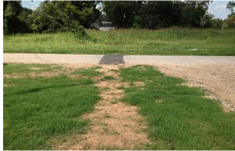
The project included connections to existing services and pavement repairs.
