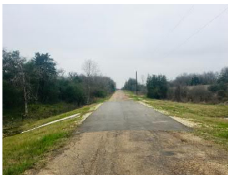
Completed concrete culvert and asphalt pavement repair.
