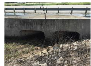
Existing 6-foot by 4-foot box culverts under FM 2004 to have proposed flood gates implemented.
