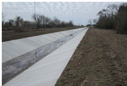
Views of the completed reinforced concrete slope paving in an existing drainage channel.
