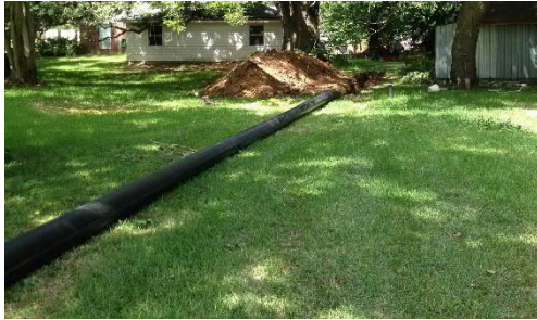
Sections of the sanitary sewer pipe went through residential areas.
