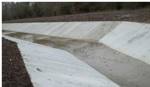
Views of the completed reinforced concrete slope paving in an existing drainage channel.
