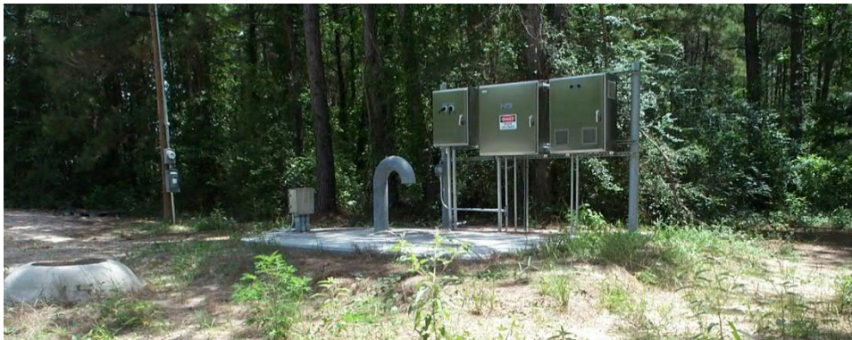
New Splendor lift station to serve approximately 120 homes.
