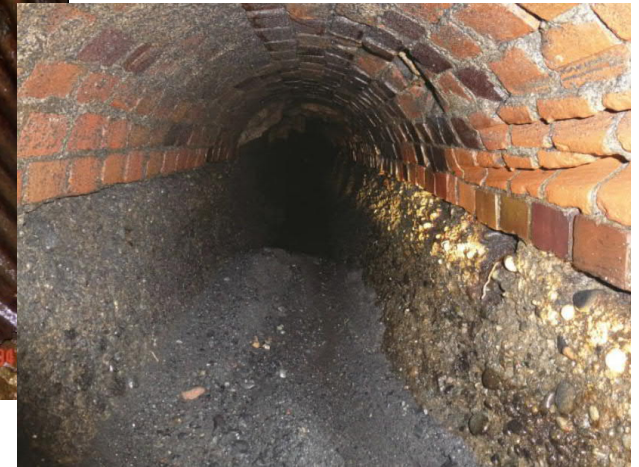
Typical Brick Sewer Televising Footage
