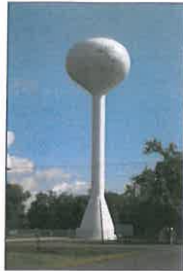
Galveston County WCID No. 8 New Elevated Storage Tank
