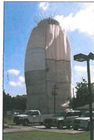
Galveston County WCID No. 8 Elevated Storage Tank Rehab
