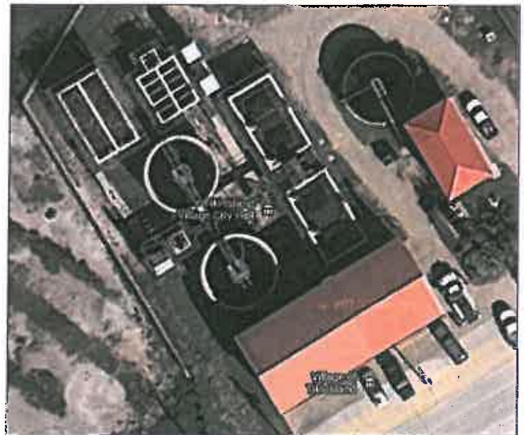
Galveston County FWSD No. 6 WWTP
