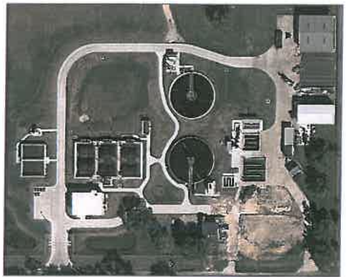
Galveston County WCID No. 8 WWTP
