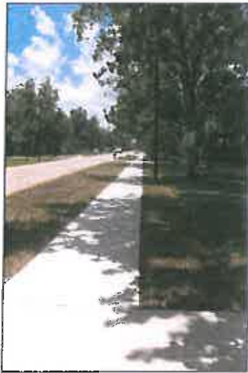
City of Richwood Enclosed Ditch with Sidewalk
