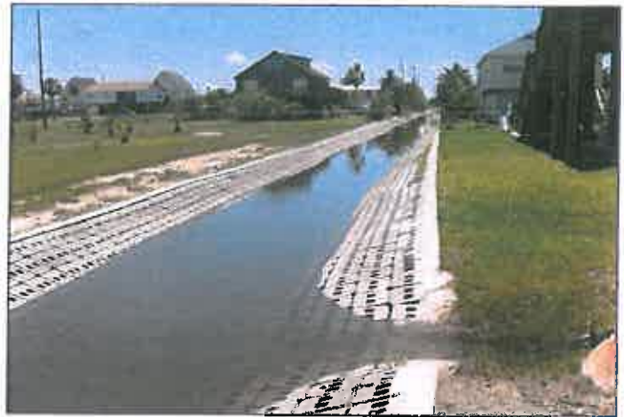
Jamaica Beach Drainage Outfall
